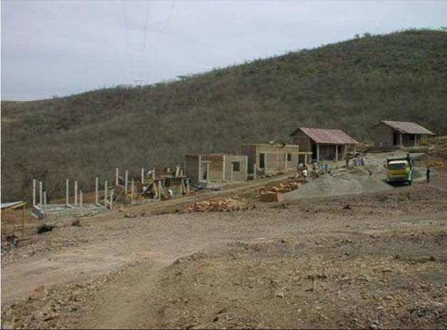
Construction of houses in Comayagua in a production line approach with different activities following each other
