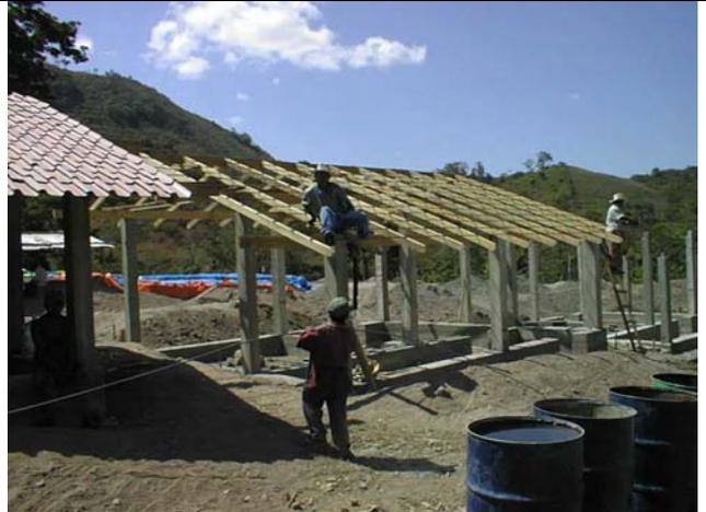
Roof construction preceded wall construction so that adobe could be stored under cover and so that walls could be built even in wet conditions
