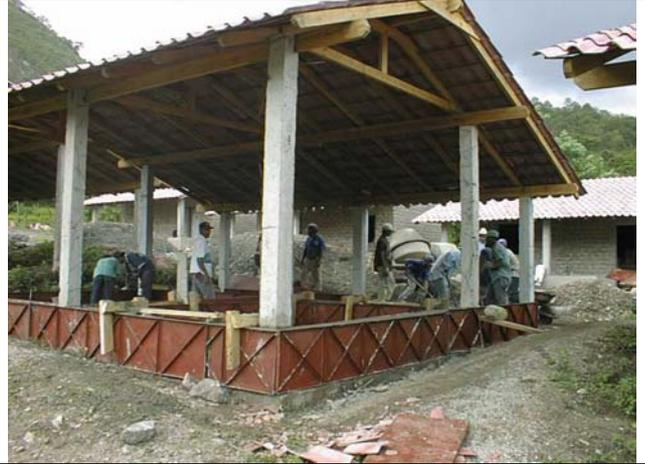
Ground beam construction carried out with formwork used in every house to speed construction
